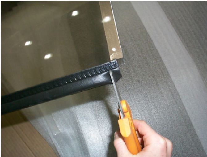
Fig. # 6 Cut the seal at the marked location
