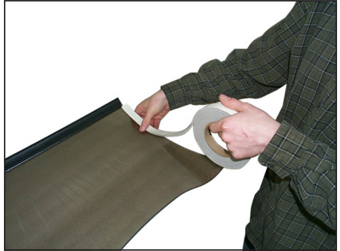
Fig. # 2 Install vinyl foam
