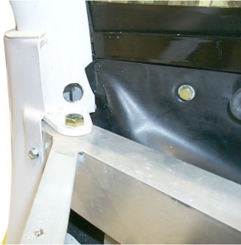
Fig. # 12 Drill lower hole in roof rail
