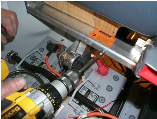
Fig. # 3 Disconnect license plate lamp ground wire
